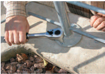
Fixing of railing
